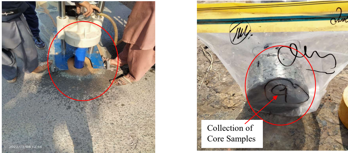
Figure 4: Collection of core samples of rut prone roads
